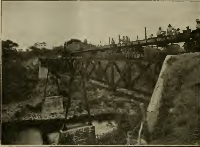
RIO MAJAGUA BRIDGE—CHIRIQUI NATIONAL RAILROAD.
